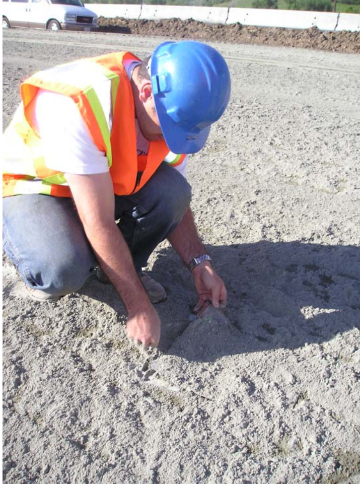
FIGURE 3.6 Retrieving cement collection sheet.
