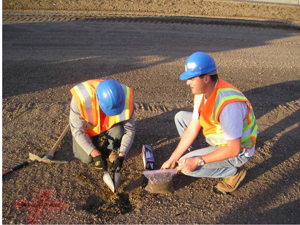
FIGURE 3.4 Sampling base material before cement placement.
