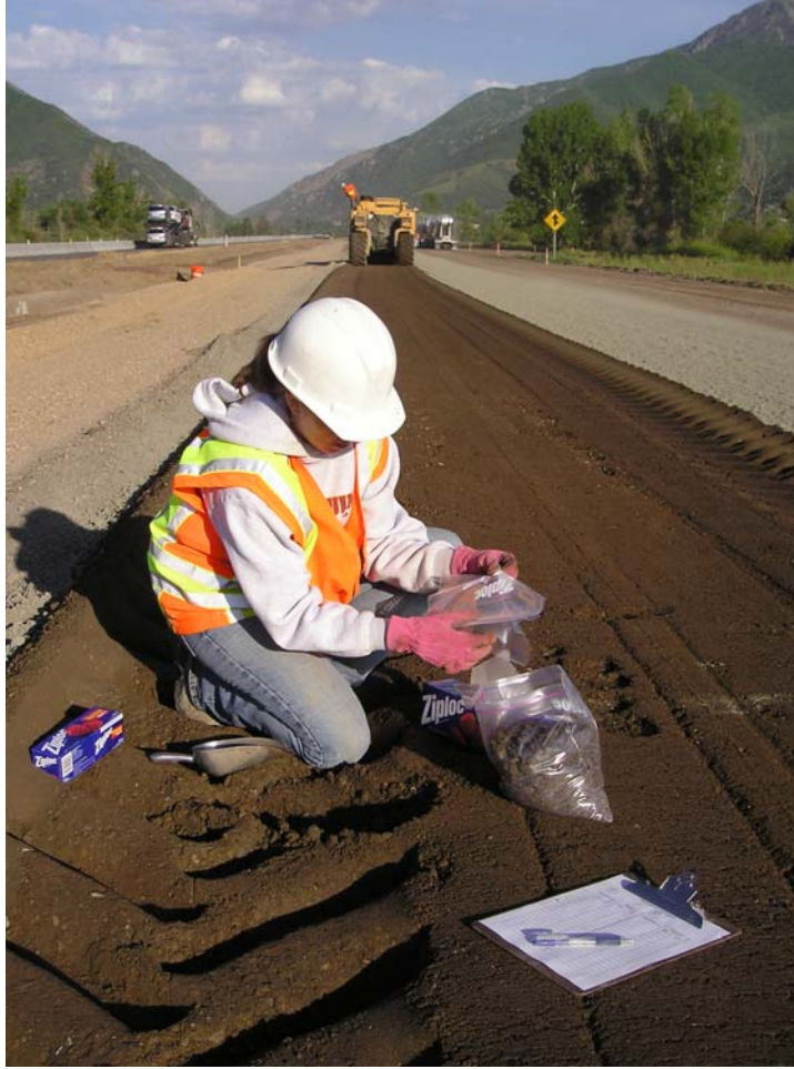
FIGURE 3.8 Sampling base material after cement mixing.
