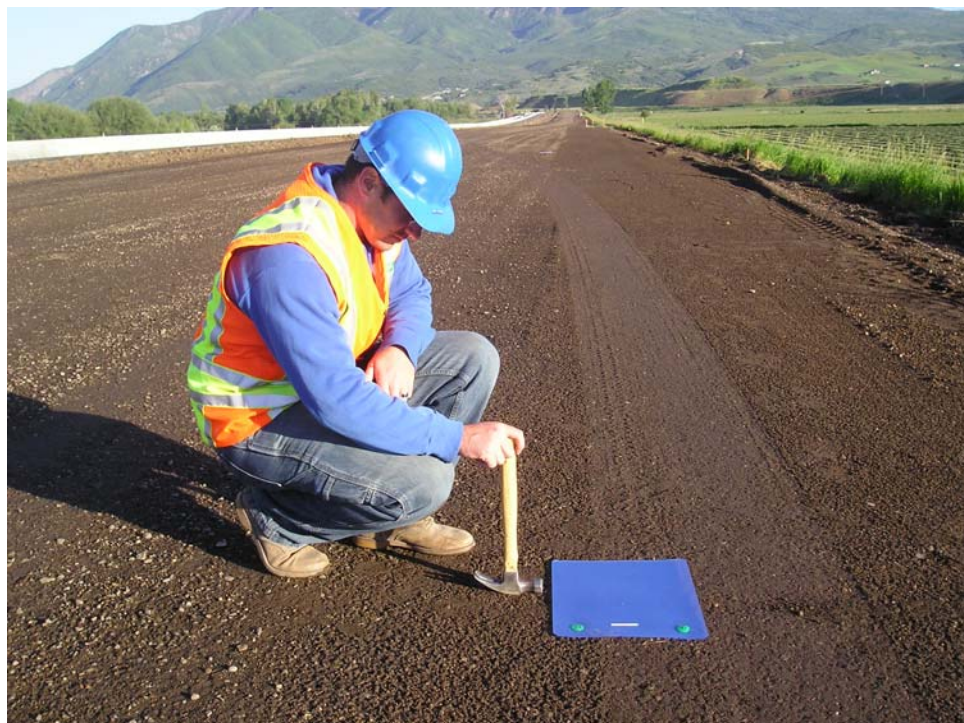
FIGURE 3.5 Placing cement collection sheet.
