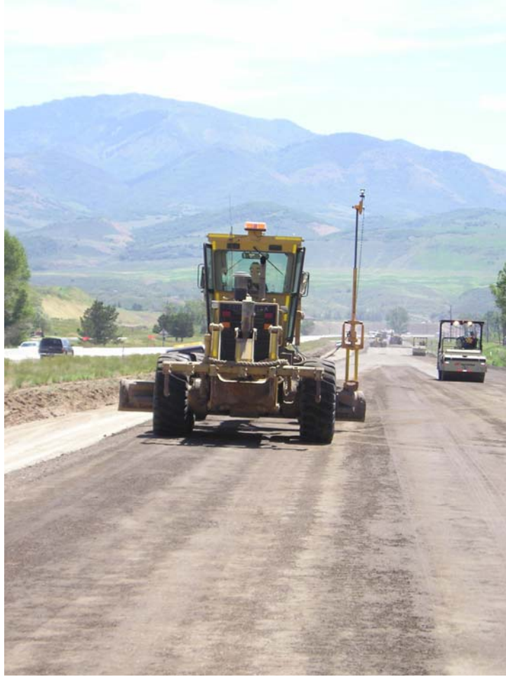
FIGURE 2.6 Grading process.
