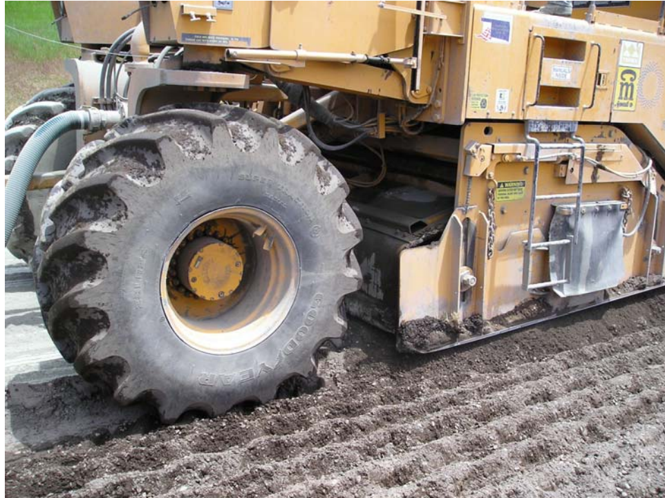
FIGURE 2.3 Cement mixing process.
