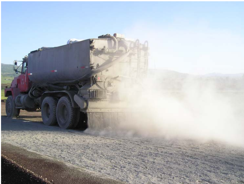
FIGURE 2.2 Cement placement process.
